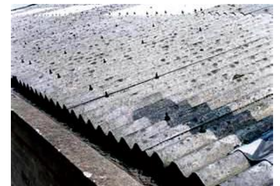
ASBESTOS ROOFING & BOARDS
